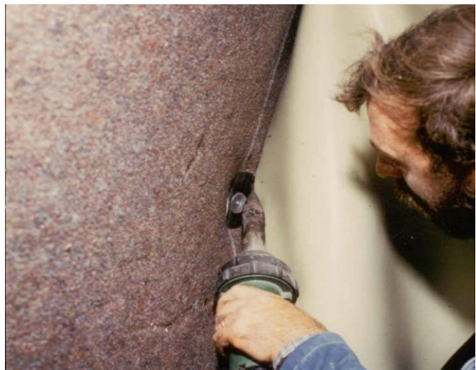
Fixation of the geomembrane by spot welding
