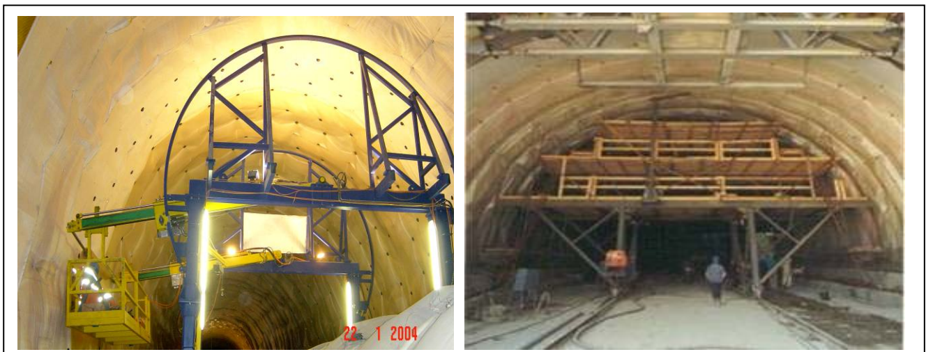
Hydraulic scaffolding on wheels
