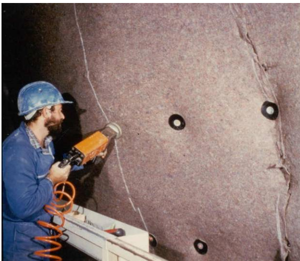
Fixation of the geotextile
