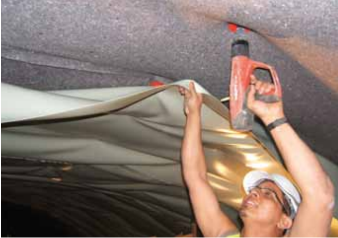
Fixation of the geotextile
