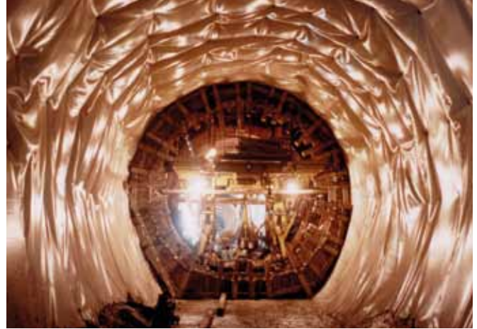
Fixation of the geomembrane by spot welding
