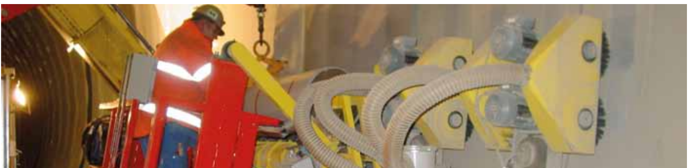
Installation geomembrane with glue
