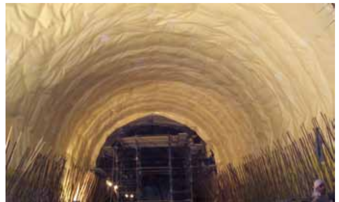
Scaffolding for manual installation
