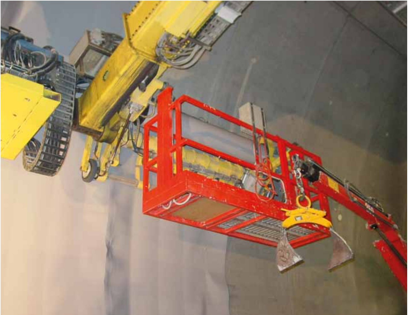
Installation geomembrane with glue
