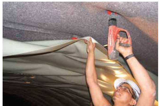
Fixation of the geotextile
