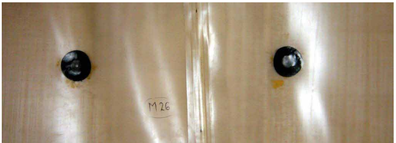
Fixation of the geomembrane by spot welding
