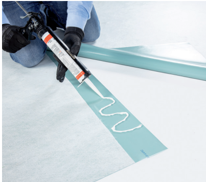
Sealing by mastic glue RENOLIT CEM 805 .
