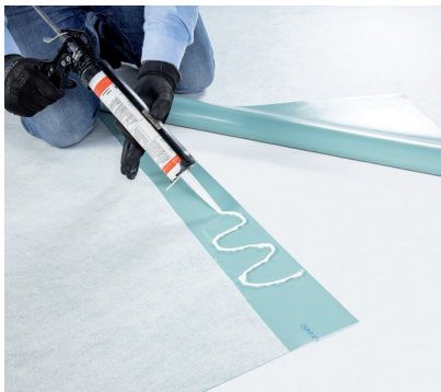
Sealing by mastic glue RENOLIT CEM 805 .
