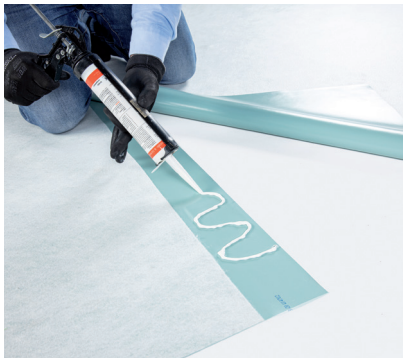
Sealing by mastic glue RENOLIT CEM 805 .
