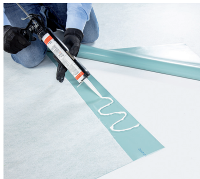
Sealing by mastic glue RENOLIT CEM 805 .
