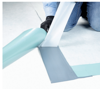
Butyl tape sealing for transversal overlap.
