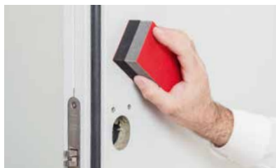
2. Prepare the surface
