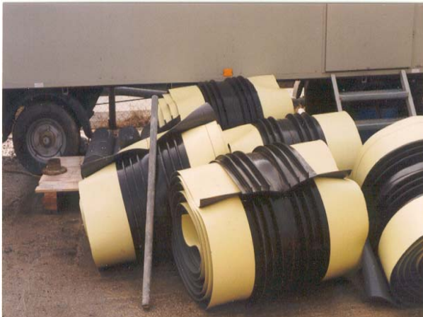
Geomembranes with welded water stops produced in prefabrication
