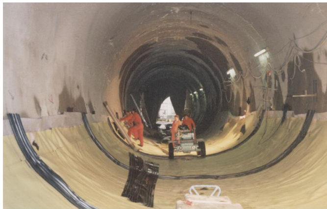
Water stop of bottom slab
