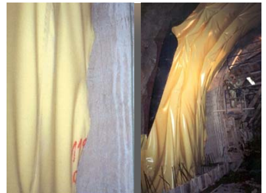
Head shuttering of the concrete unit
