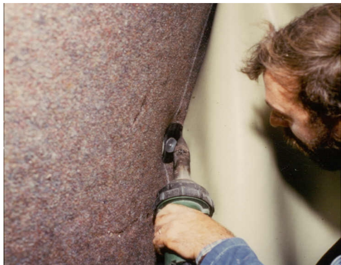
Fixation of the geomembrane by spot welding
