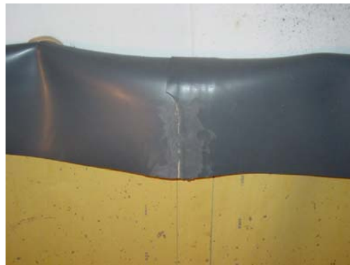
Prepared seam for T-cross
