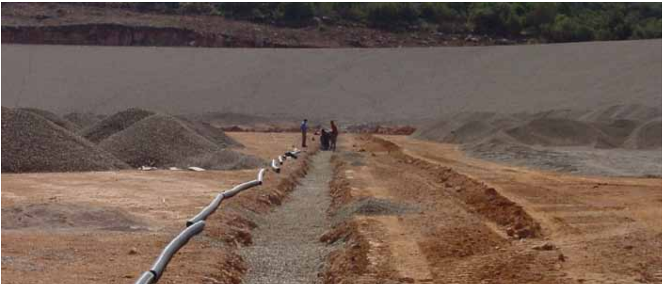
Drainage pipes under waterproofing
