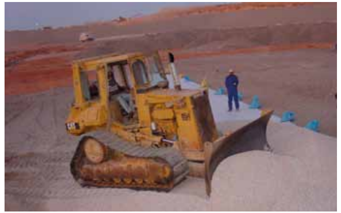
Distribution of material with bulldozer
