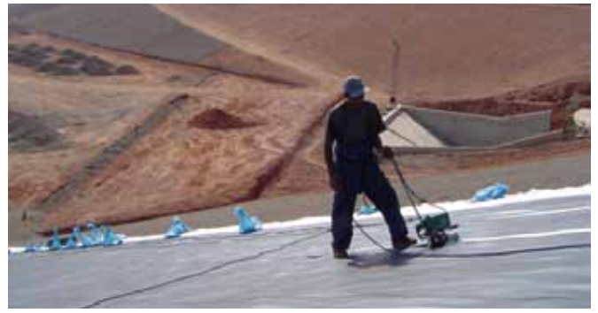
Welding with hot air and double seam
