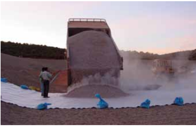
Unloading of protection material with truck
