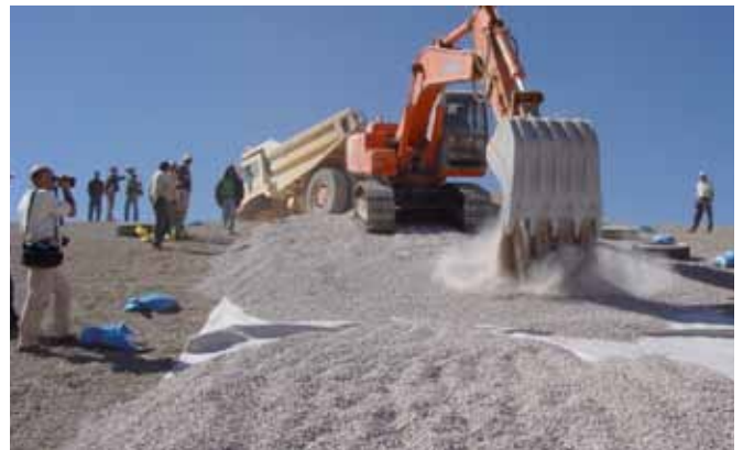
Distribution with excavator
