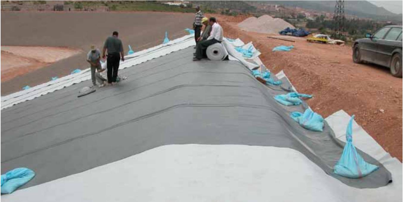
Welding with hot air and double seam
