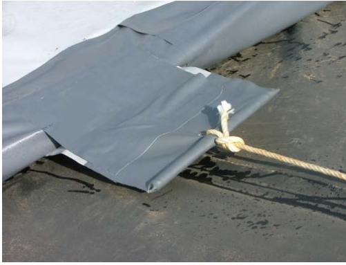
Loops for pulling the floating cover
