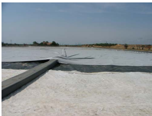
Installation floater under floating cover
