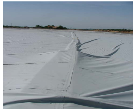
Installation floater under floating cover
