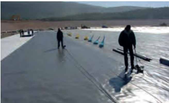
Welding of the geomembrane
