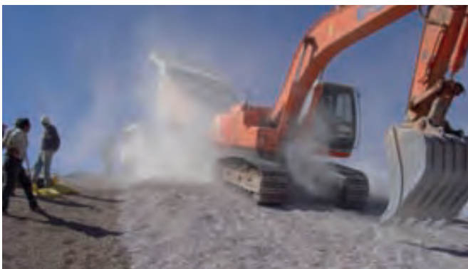
Placing of the upper drainage layer
