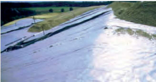
Protection layer with drainage gravel
